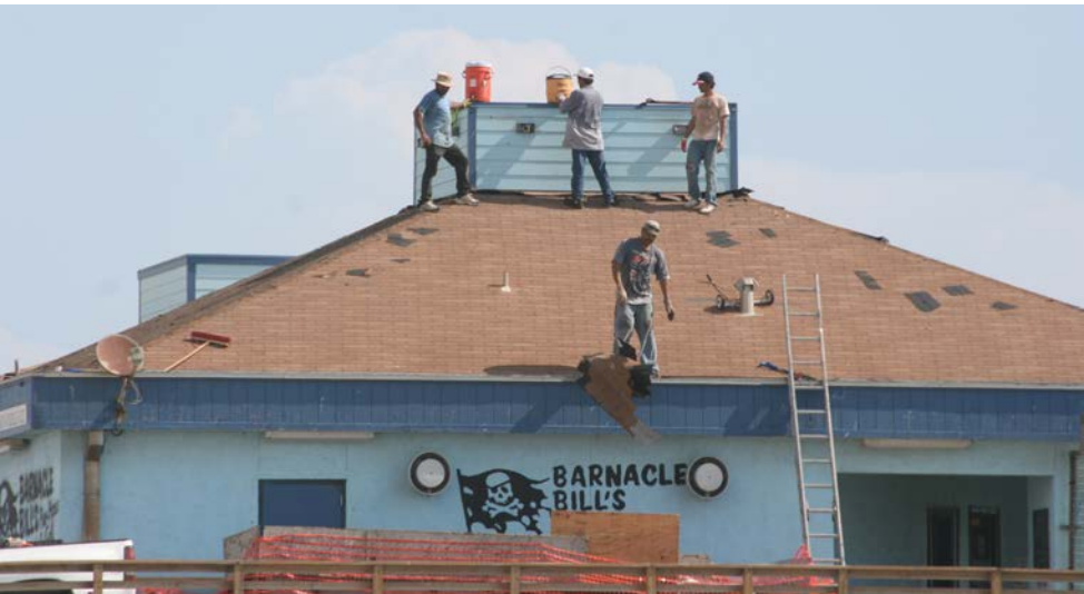
The restaurant building at Bob Hall Pier was under construction.
