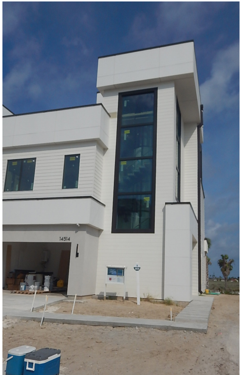
Work on the model homes at Whitecap NPI is winding down and expected to be finished by the end of the year.
