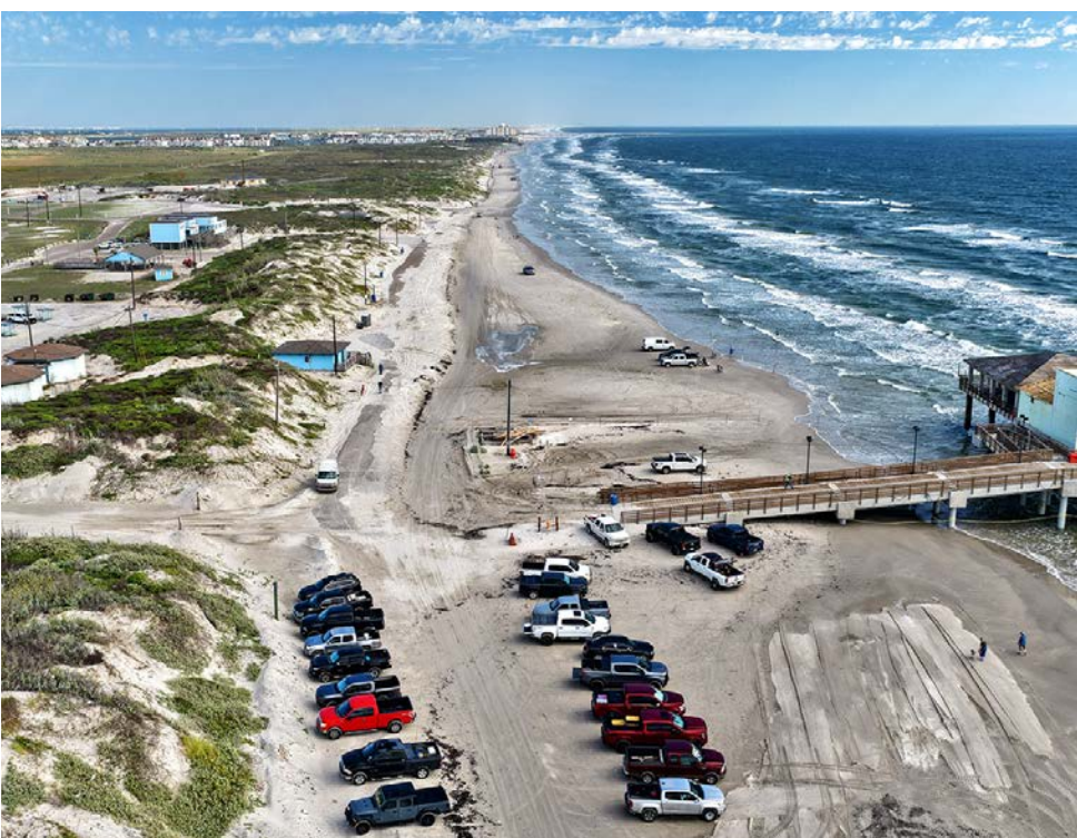
Construction on the road from Billy Sandifer Way to Bob Hall Pier previously scheduled for September has still not begun. The work has been delayed to prevent damage from heavy equipment during construction on Bob Hall Pier, and will begin by the end of the year.
