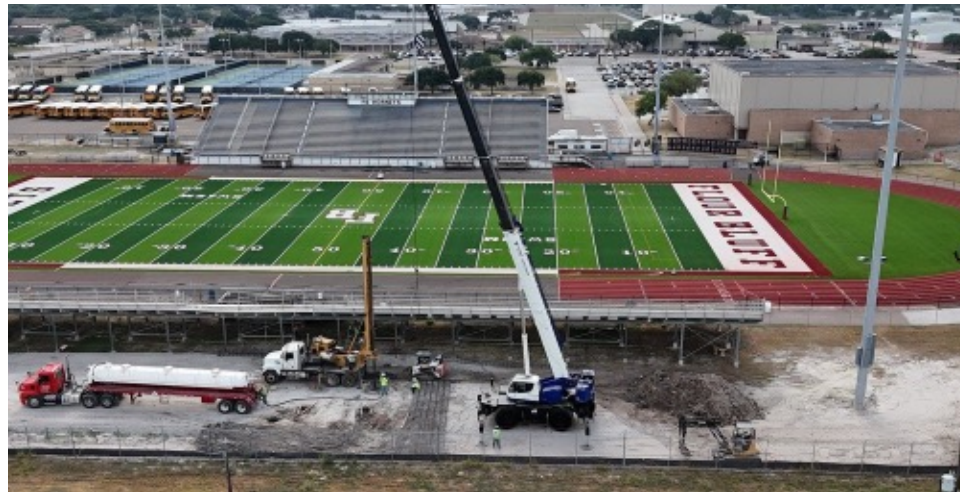
Current progress on stadium construction
