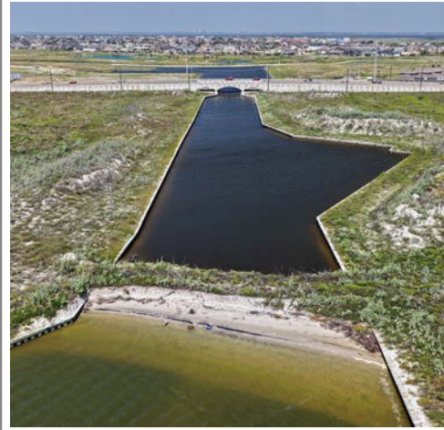
The Don Patricio Bridge and the Sand Dam
