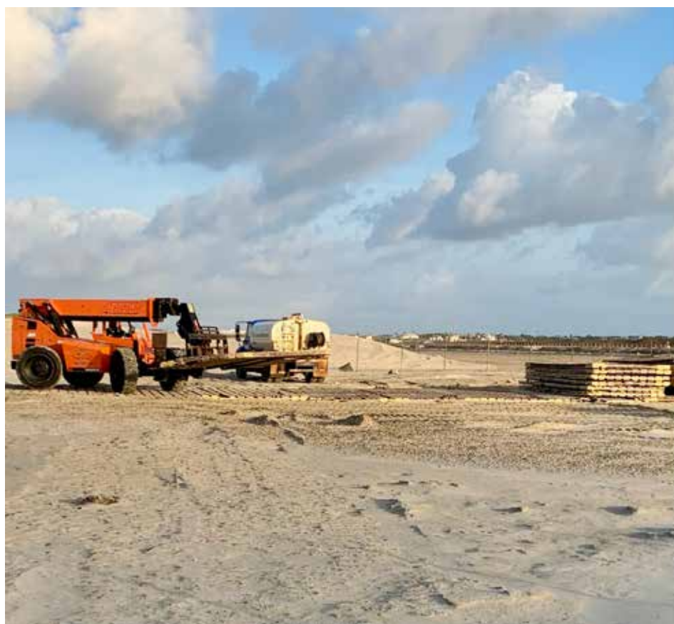
Work on Packery Jetty repairs began in the yard this week. Photos by Evelyn Pless-Schubert.
