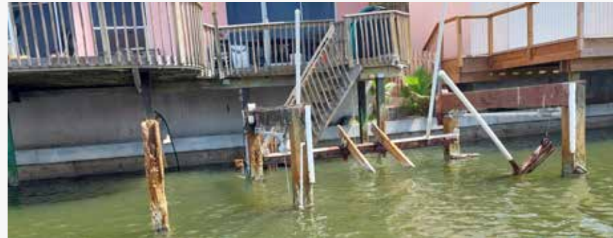
This is what the PIPOA Canal Boat is looking for. Obviously, it is a potential danger in a storm and a danger to boaters when pieces float away.
