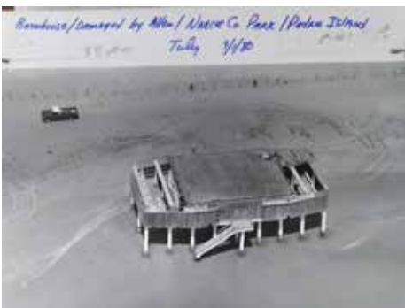
The boathouse at Nueces County Park after Hurricane Allen. Photo taken September 1, 1980 courtesy of Caller-Times.
