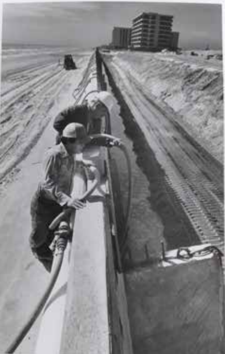
Reconstruction of the Michael J. Ellis Seawall after damage from Hurricane Allen. Workers Joe Hernandez and Santos Garcia (rear) handle hoses which will attach to pipes which will pump water to the base of the seawall in an attempt to settle the seawall structure back into place. Work was done by Padre Isles Construction. This photo courtesy of the Caller-Times dates February, 27, 1981.
