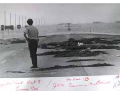
Where the trouble started. This shot was taken as Hurricane Allen approached. It shows the water covering the road, which was the evacuation route, from the north side of the barriers. When the incoming tide overtopped the barriers they fell unleashing a torrent of water that found its way into the Island canal system. Photo courtesy of the Caller –Times. Picture 4 shows the submerged roadway after the barriers were swept away.
