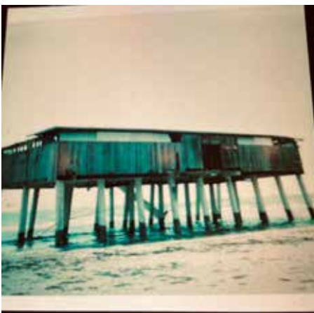
Cabins near Bob Hall Pier after Hurricane Allen.
