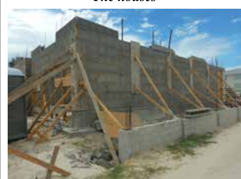
ICF house currently under construction in Port Aransas.
