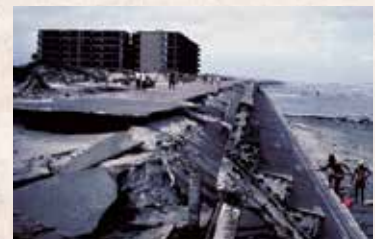
The Michael J. Ellis Seawall sustained "some damage" according to the Padre Isles Property Owners Association.
