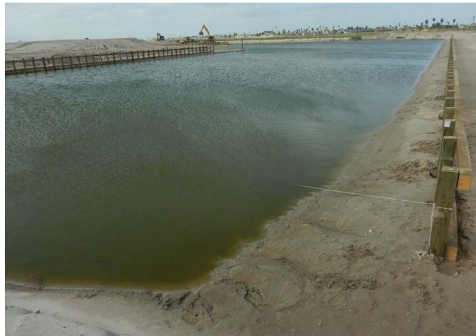
The bulkheads on the west side of the Don Patricio Bridge are now under construction. The first bulkheads were removed to widen the channel after plans changed. The original plans called for retail and office space on the south side of the channel, but the channel was widened to allow for the location of a marina, dry stack boat storage, and yacht club there. The north side of the channel (right) will include retail and residential space but final plans are not yet complete.
