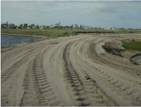
This berm of sand will be removed when the channel under the new bridge is opened to connect the six miles of newly dug canals on the Whitecap NPI site to the existing Island canals and saltwater in the next few months.
