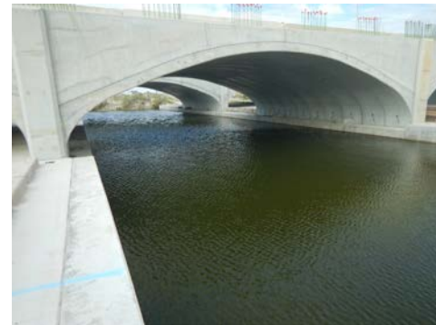
The clearance from the water to the center arch of the bridge is 14 feet.
