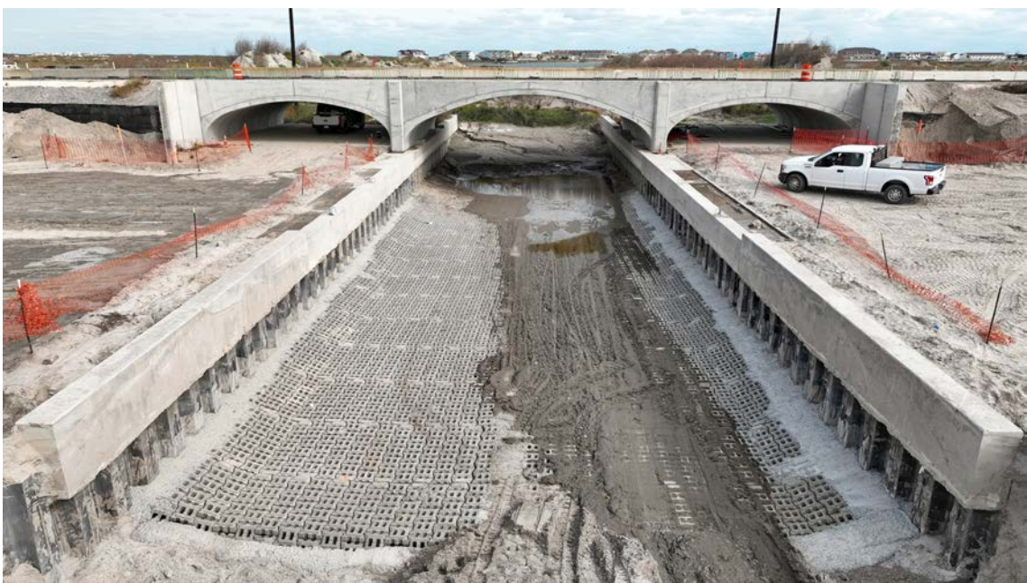
Crews this week began work to line the bottom of the channel under the Water Exchange Bridge under construction on SPID. The blocks seen here are designed to harden the floor of the eight-foot deep channel to prevent erosion.
