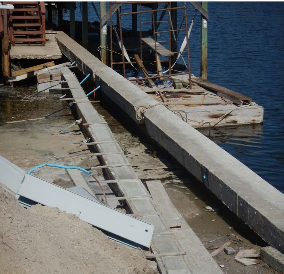
Work to stabilize the damaged bulkheads after TS Alberto.
