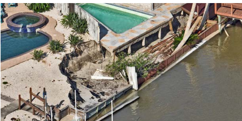
Bulkhead damage from Tropical Storm Alberto
