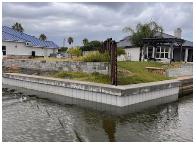
Repaired bulkheads in the Island Canals
