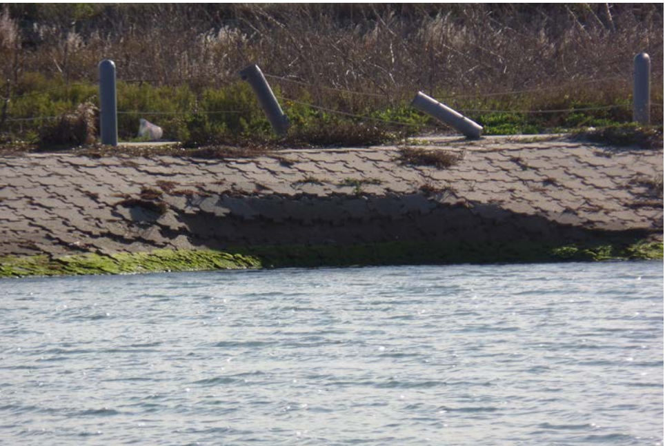
Even before Hurricane Harvey, the walls along Packery Channel continued to collapse and were in need of repair. City money was used for the repairs, part of which was refunded by FEMA
