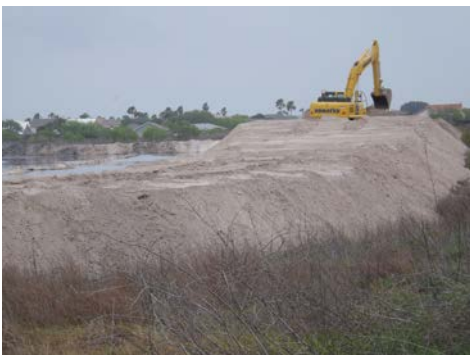
Sand from canal dredging was being pumped to this site near Aquarius.
