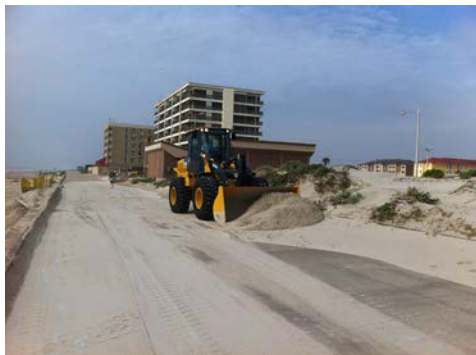
Sand was being plowed from the Micheal J. Ellis Seawall
