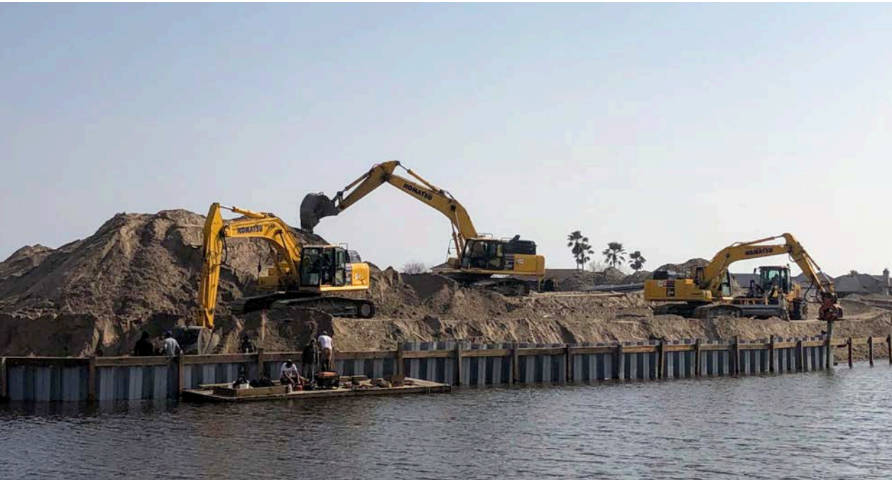
Installing the bulkhead infrastructure at Whitecap NPI.
