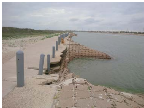
The damage to the Packery Channel Jetties now under repair was caused by Hurricane Harvey in 2017.
