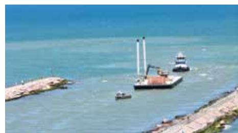
Barge to repair more Packery Channel jetties arrives.
