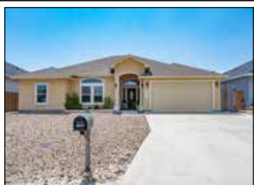
15810 Gypsy St. Beautiful 3/2/2 @ 2127 sq. ft. Well landscaped with in-ground concrete pool! Call Randy Corpuz 361-765-9914
