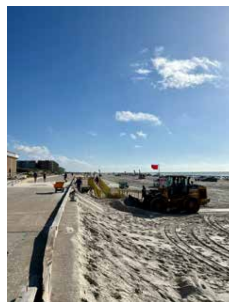
CC Beach Operations removed blown up sand at the parking lot, seawall, ramps and beach showers.
