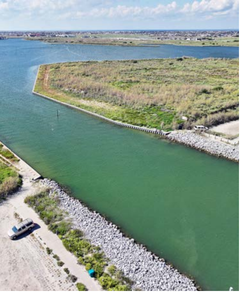
The current state of the old seagate area with Lake Padre in the background
