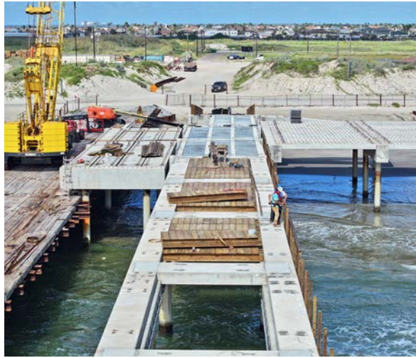
At Bob Hall Pier the pilings are in place and concrete walkways are being installed with completion expected by the end of 2025. No contract has been announced for a construction firm to build the new restaurant facility at the pier.
