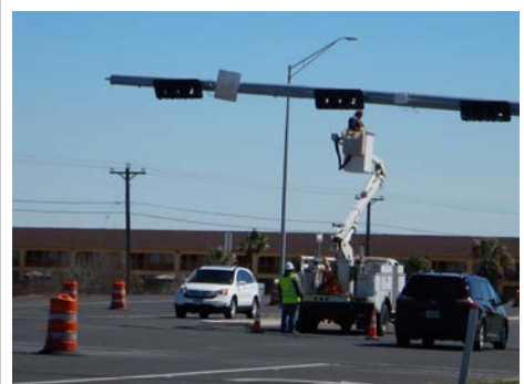
Traffic light at Aquarius being installed in 2016
