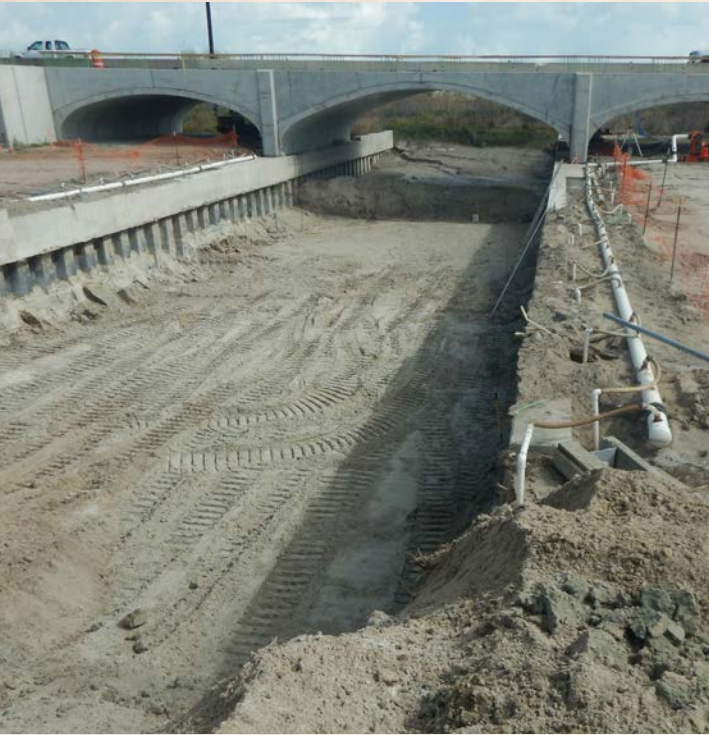
Crews this week began digging the 8 foot deep channel under the WATER EXCHANGE BRIDGE
