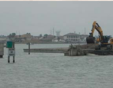
In early 2022 crews began demolition work on the sea gate opening between Lake Padre and Packery Channel to widen the entrance to about 75 feet.
