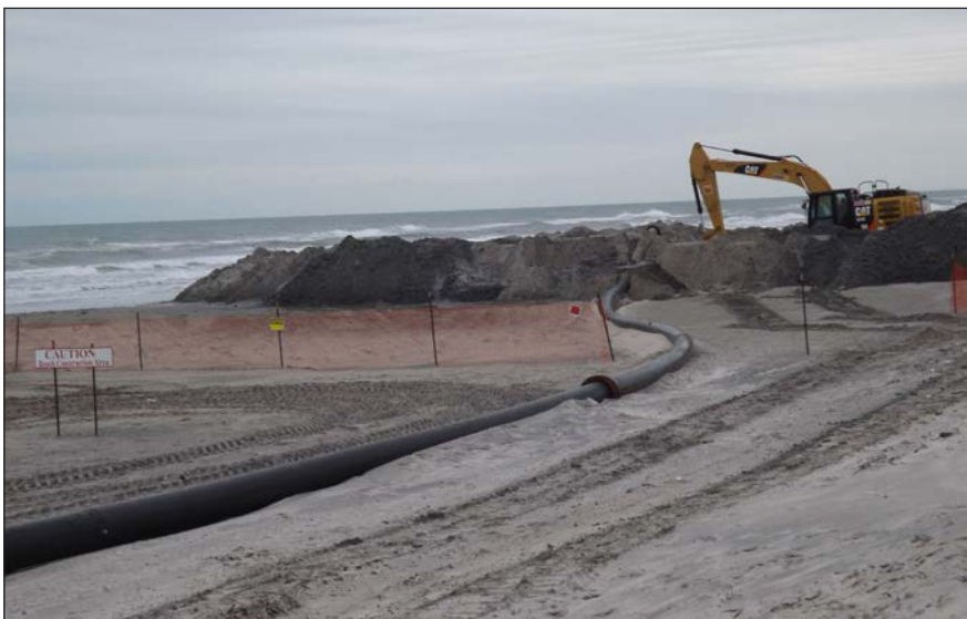
Packery Channel was being dredged and the sand used to widen the beach.
