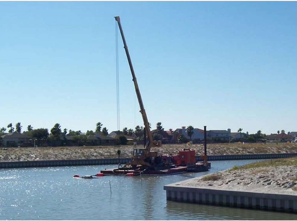
Dredging continued in the canals around Commodores Point
