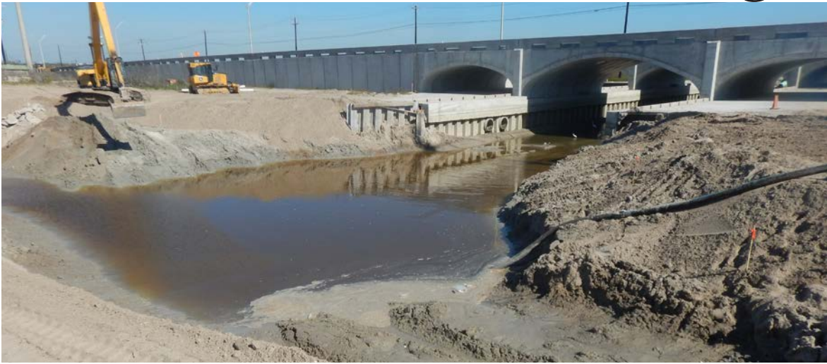
Crews are moving the sand dam on the west side of the bridge further from the bridge structure in order to place articulated mats along the canals next to the bridge for scour protection.
