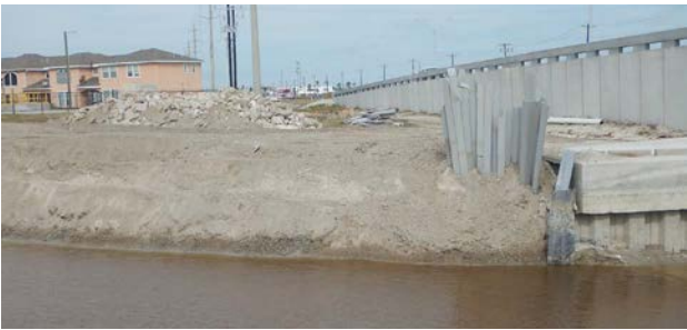
Crews are working to armor the approaches to the Don Patricio Bridge
