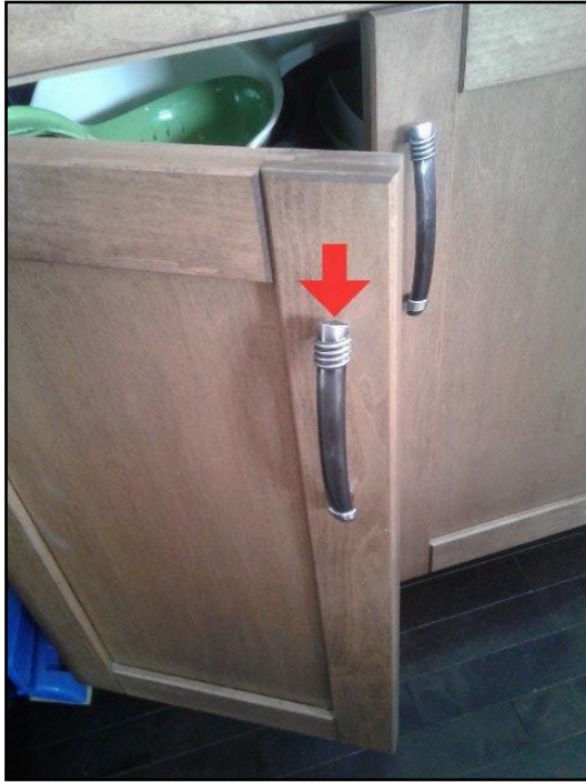
34. Pieces missing or loose
