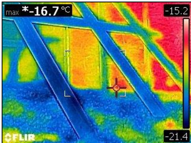
48. Area Noticed from Attic
