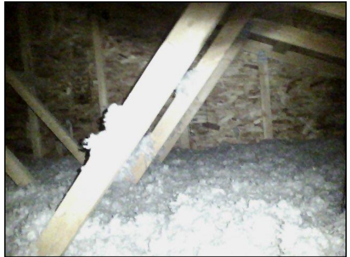
49. Area Noticed from Attic
