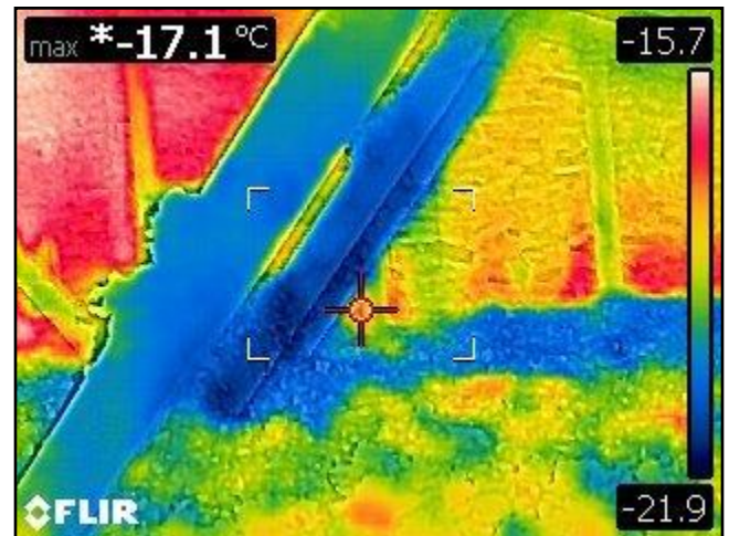
47. Area Noticed from Attic
