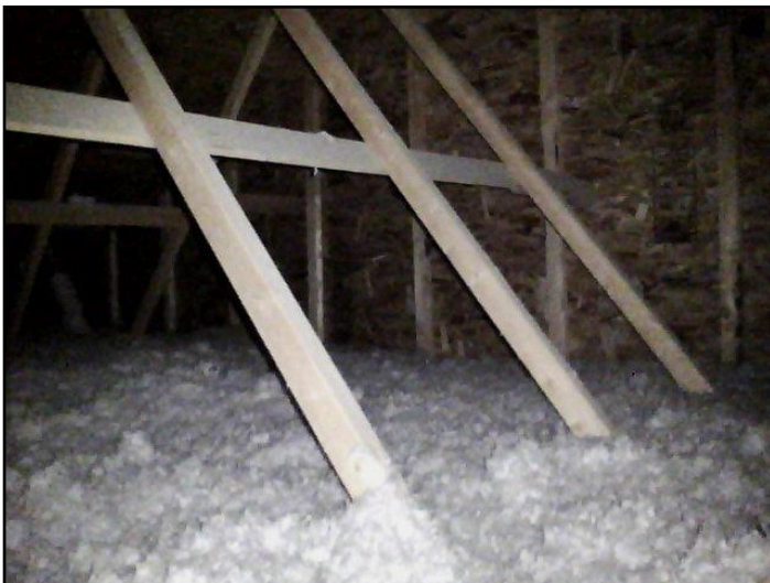
42. Area Noticed from Attic
