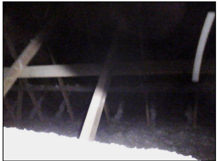
45. Area Noticed from Attic
