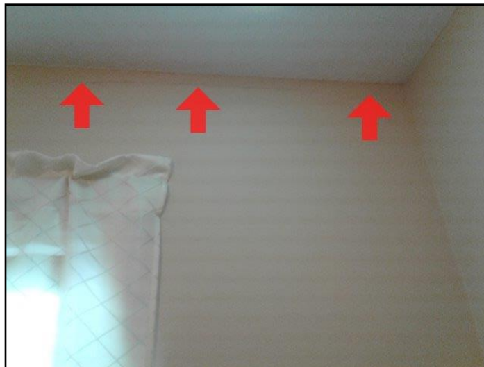
33. Poor joints
