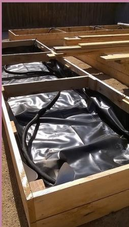
Putting in the liner. If the ground is rough, it is recommended to add a layer of sand or fabric on the bottom before putting the liner in. It is also recommended to add another layer of fabric on top of the plastic at least to the depth of the rocks to avoid them puncturing it. This step can be left out if using an IBC.
