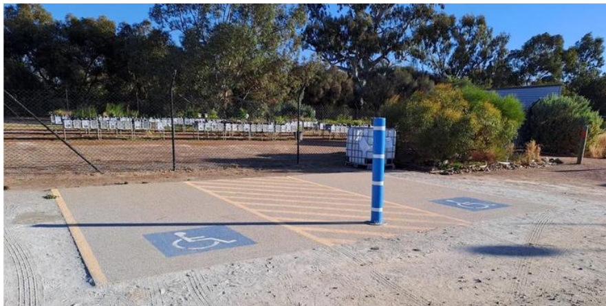
Photo 2: Disability Car Park at the Community Nursery
