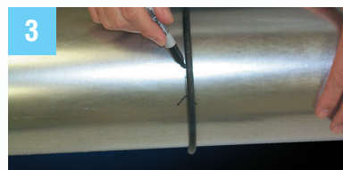
3 Use O-ring provided and mark for cut.
