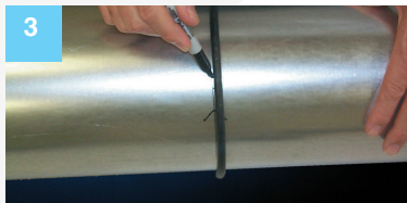
Use provided O-ring to mark for cut.
