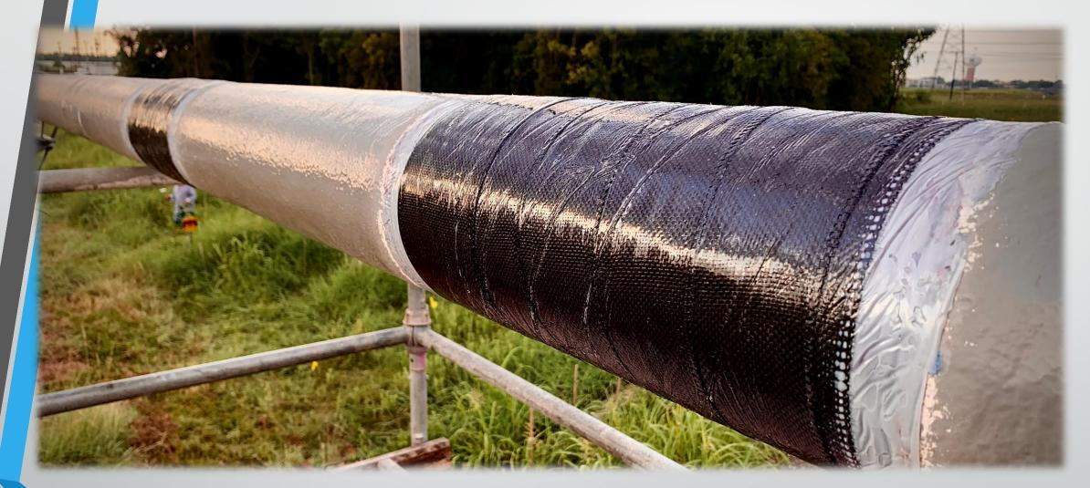
DOT, PHEMSA, ASME PCC-2 and ISO 24817 compliant Engineered Composite Wraps
