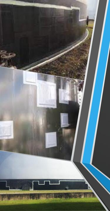
As of June 2020, the API 653 standard now includes allowances for the use of composite repair patches on the shell of a tank.
