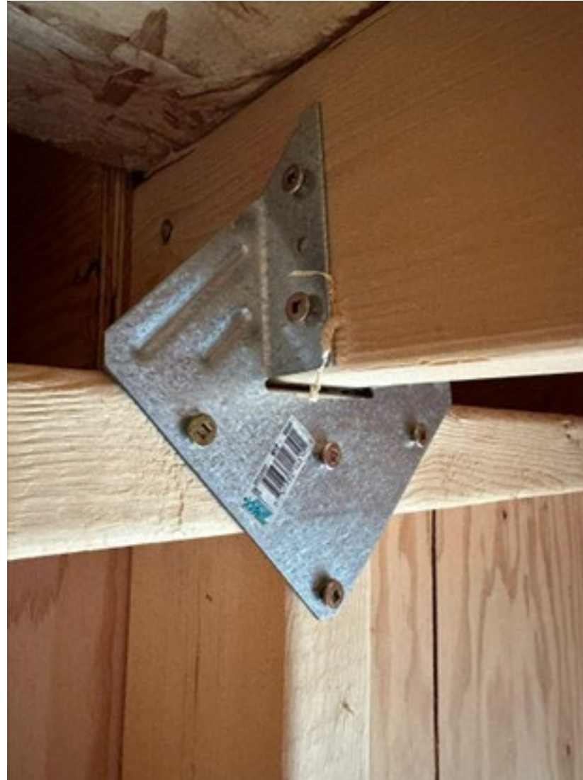
Figure 2.3: Metal hurricane tie attaching ceiling joist to wall frame
