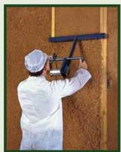
**STEP ONE:** A unique spray-applied application in walls, floors, or ceilings that fully insulates around plumbing and wiring, reducing air infiltration and creating a comfortable environment.
