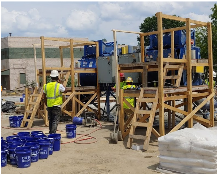
Photo: ceEntek's Model 30 Mixer Pair set up on Chartiers Run
