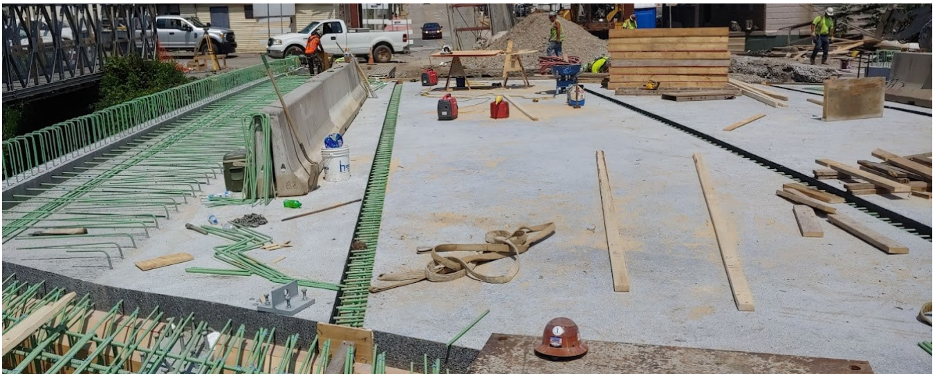
Photo: Preparation of longitudinal connections on bridge deck
