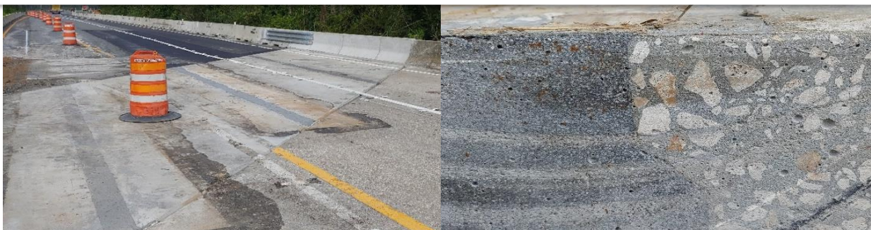
Photos: Completed approach slab connections using ce200SF-G™ (L); Close-up of the interface bond between the precast approach slab and the ce200SF-G™ cast connection (R).
