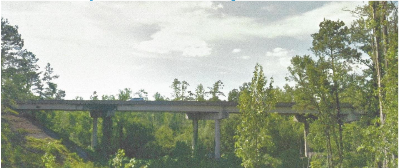
Photo: I-10 West Bound Bridge over Flat Creek, Gadsden County, Florida (Google)
