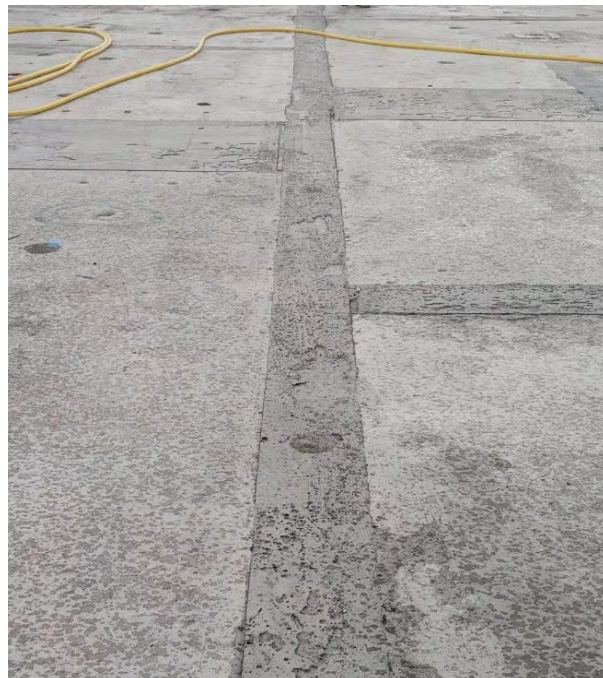
Photo: Close-up of UHPC connections (I-77 Exit Ramp).
