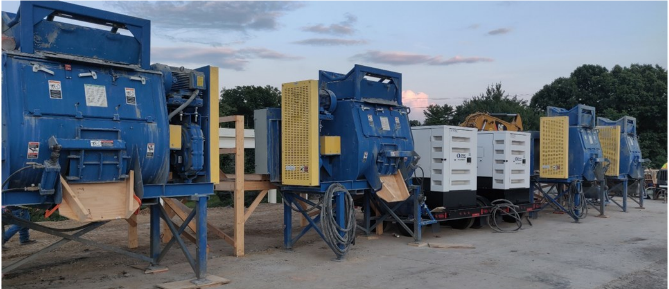
Photo: Four Mixer Set-Up for I-77 Exit Ramp
