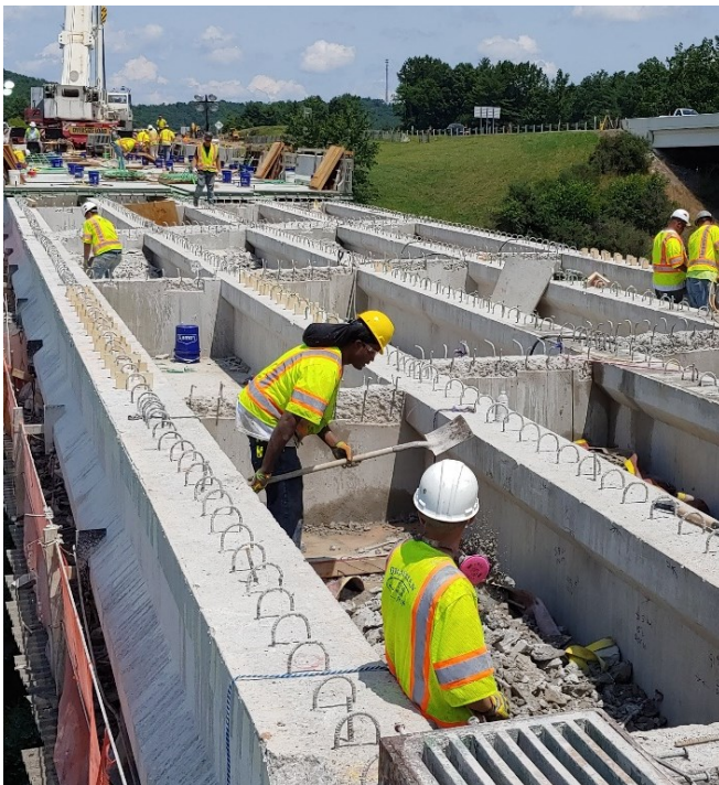
Photo: Existing precast girders (I-77 Exit Ramp)
