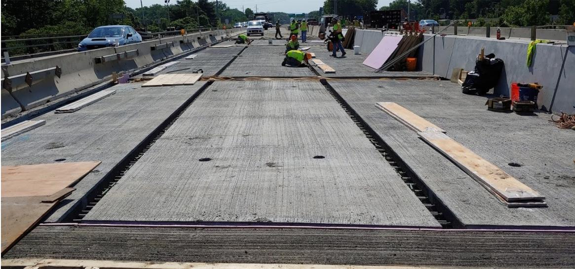
Photo: Prepping joints for UHPC on precast deck panels, I-90 over Fuller Rd, Albany, NY
