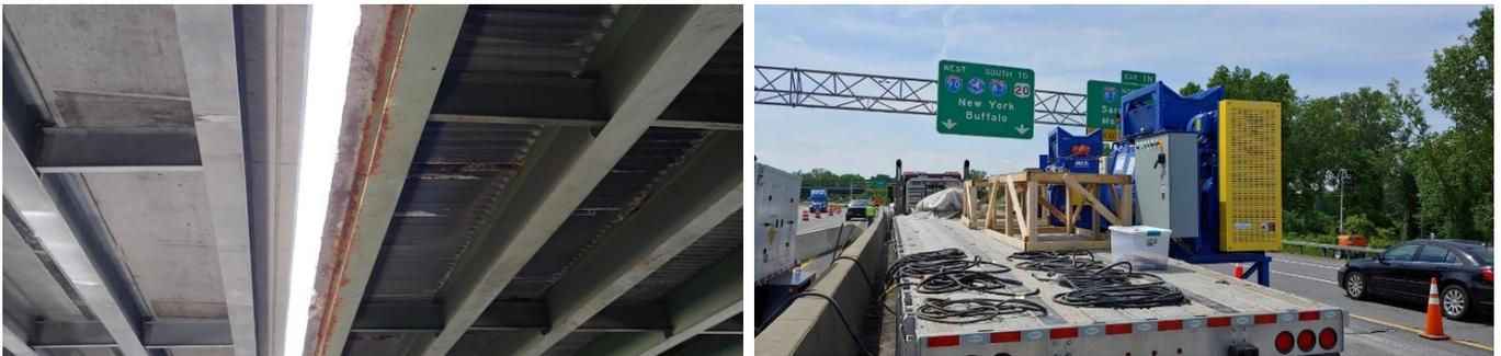
*Photos: Comparison between new and old bridge section (L), ceEntek's UHPC mixer set up in pair (R).*
