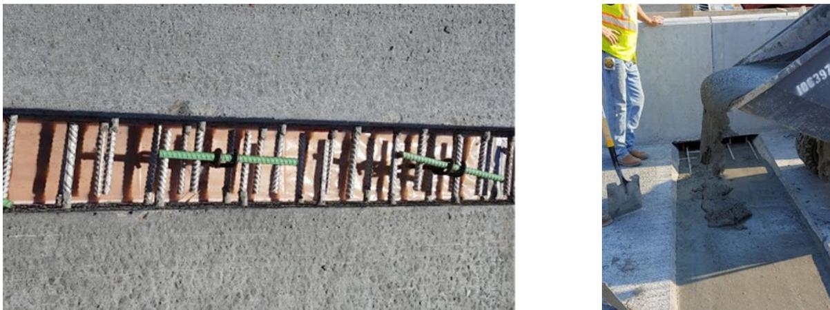
*Photos: Connection bottom formwork being prepped for casting (L), ceEntek's ce200SF-G™ being poured from power buggy into link slab (R).*
