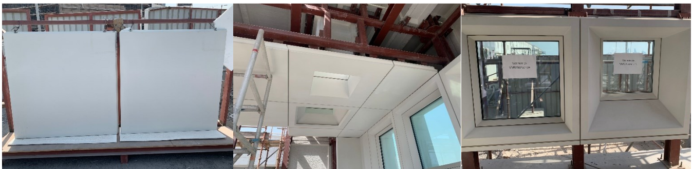
Photos: Precast UHPC Panels (L); Assembly of UHPC Panels for Podiums (R)
