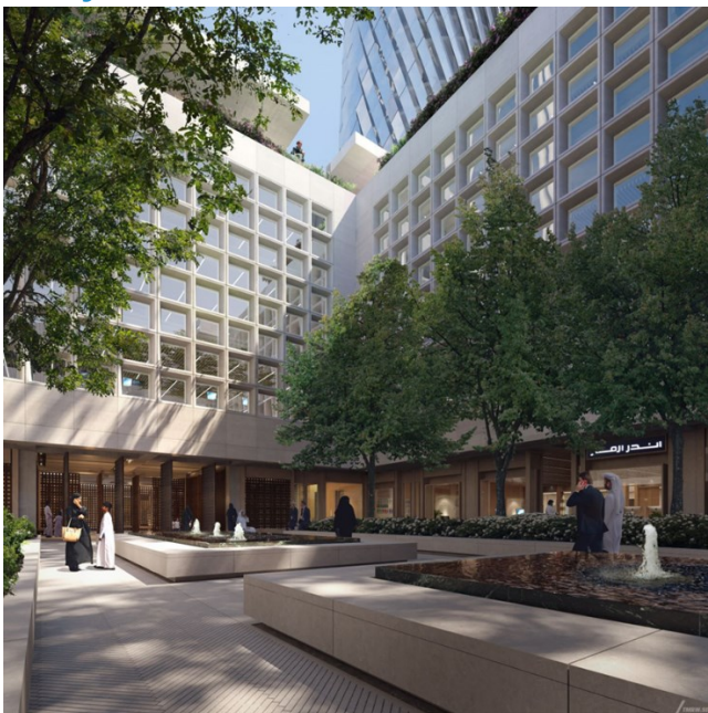
Photo: Lusail Podium Facades with rainscreen cladding
