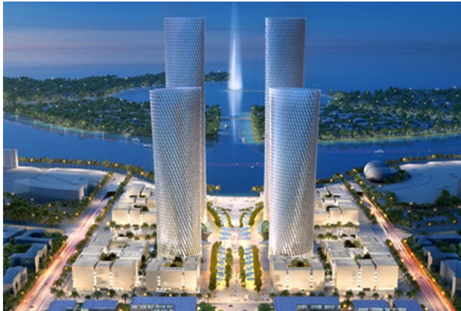
Photo: Lusail Plaza site showing the podiums with UHPC cladding (courtesy of Foster + Partners)
