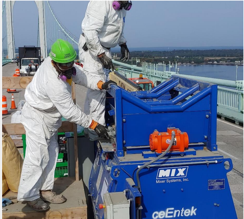
Photo: Batching of ce200SF-t™ in ceEntek's Model 30 UHPC mixer
