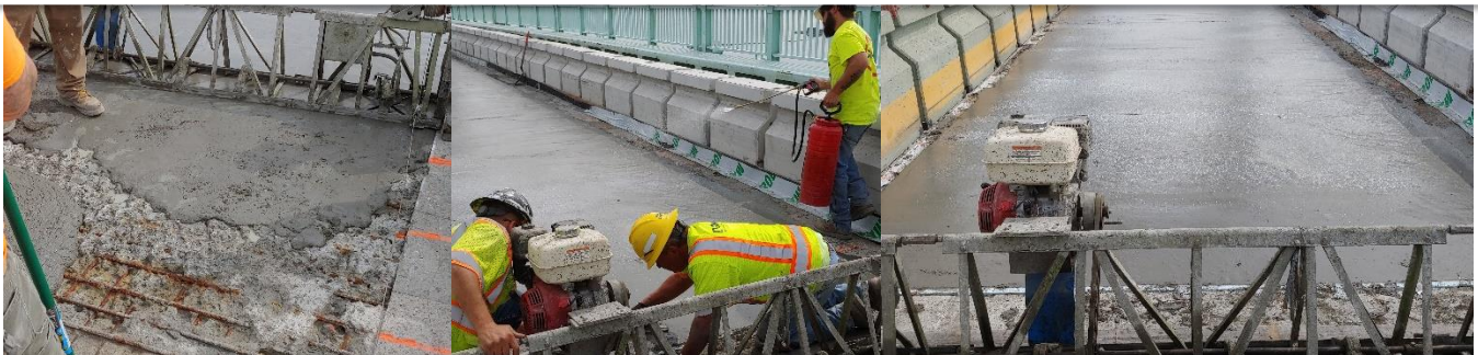
Photos: Placement of ce200SF-t™ (L); Leveling of ce200SF-t™ with vibrating screed and applying curing compound (C); Freshly placed overlay (R).
