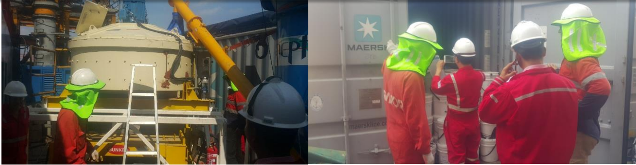
Photo: Neptune Subsea's 0.5 m 3 Pan mixer used to batch ce200-140G TM (L); Inspection of ce200-140G TM grout delivery (R)
