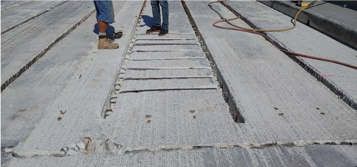
Photo: Longitudinal Connections for the Quail-Roost Drive Bridge over Canal C, Miami-Dade County, Florida
