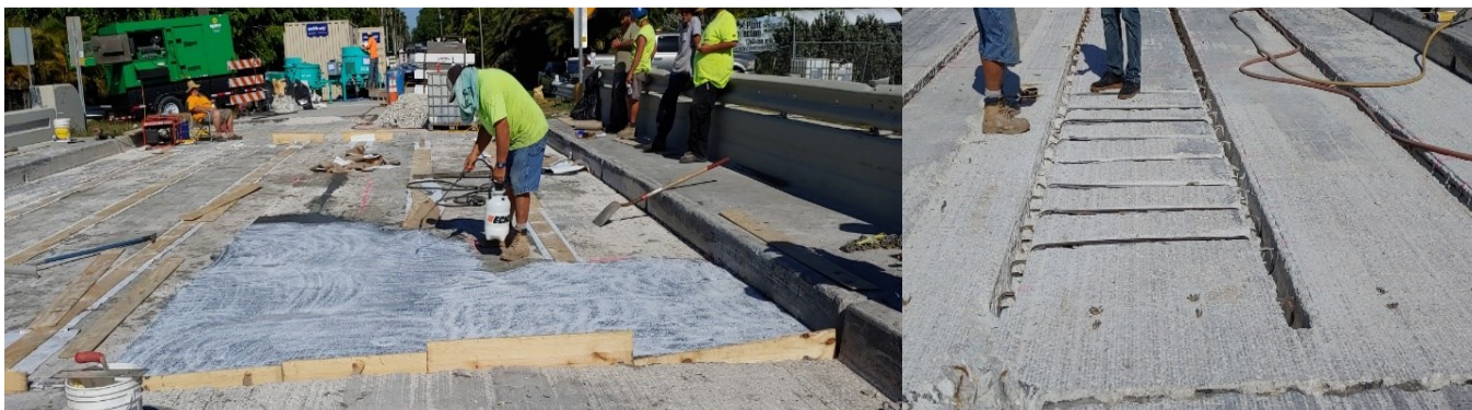
Photos: Spraying White Pigmented curing compound on the ce200SF-t™ overlay repair area (L); Close-up of the damaged area before casting the overlay repair (R).
