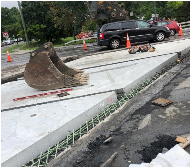
Photo: Precast Approach Slab Placement
