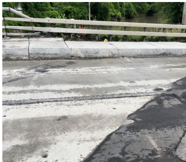
Photo: Cast Approach Slab Connection (Open to Traffic)
