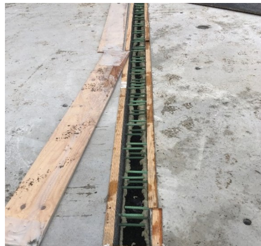
Photo: CAT MB250 Mixer (L), Prepped Connection Between Precast Elements (R)
