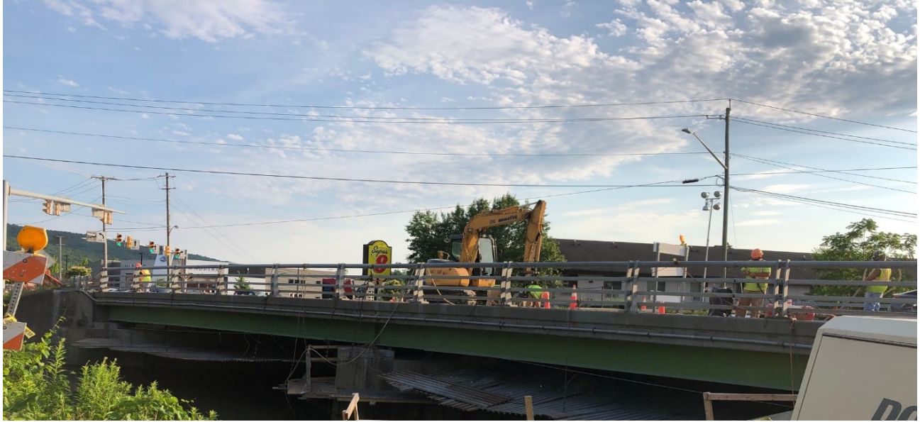
Photo: Route 13 Bridge over Mile Creek
