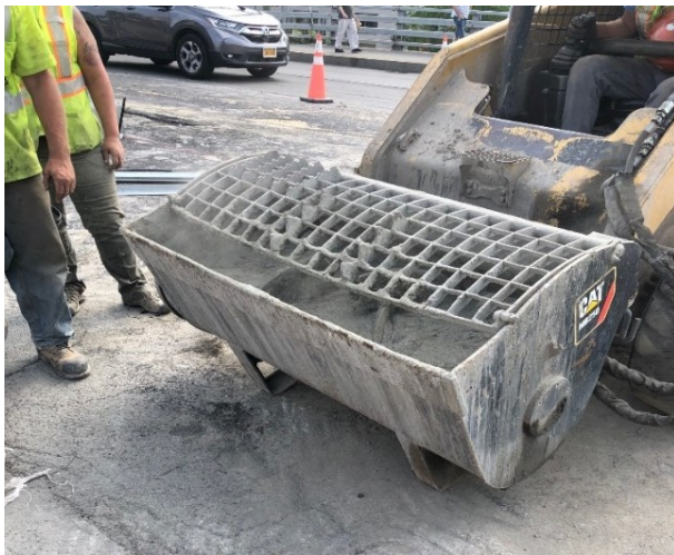
Photo: CAT MB250 Mixer (L), Prepped Connection Between Precast Elements (R)
