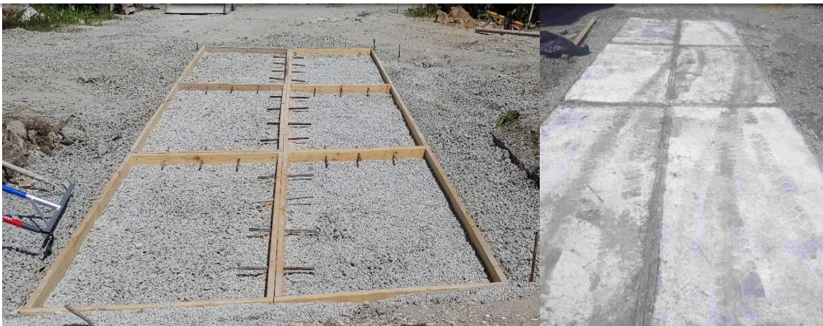
Photos: Formworks for the fork-lift ramps (upper left); completed fork-lift ramp using ce200SF-t™ (upper right)
