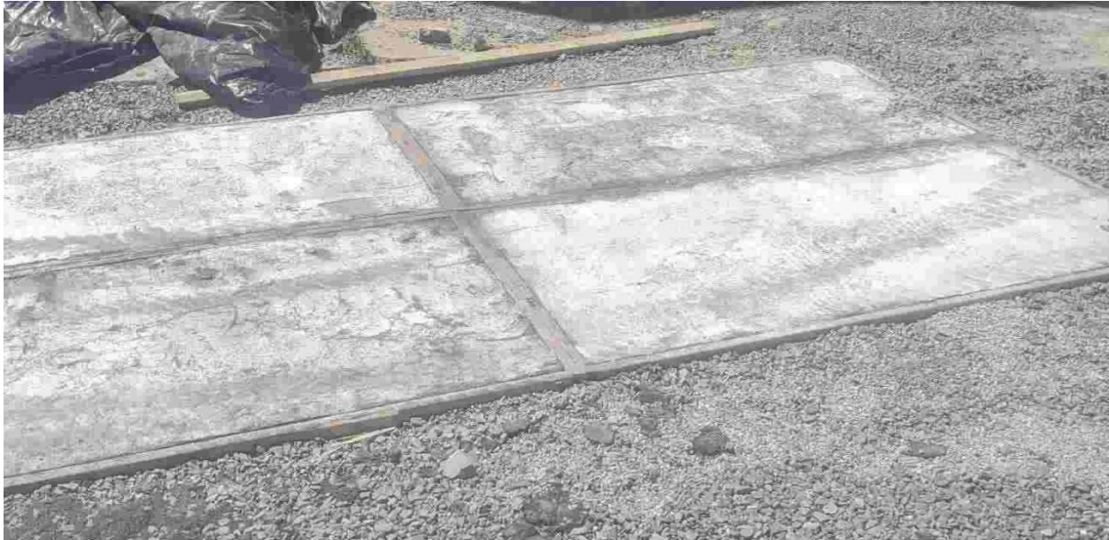
Photo: Finished ramps using ceEntek's ce200SF-t™, thixotropic Next Generation UHPC 2.0™
