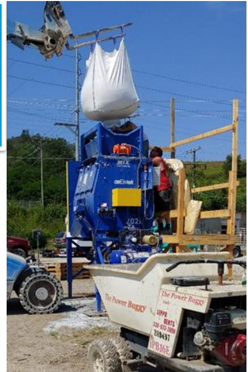
Photo: loading a bulk-bag of ce200SF-t™ into ceEntek's UHPC Mixer
