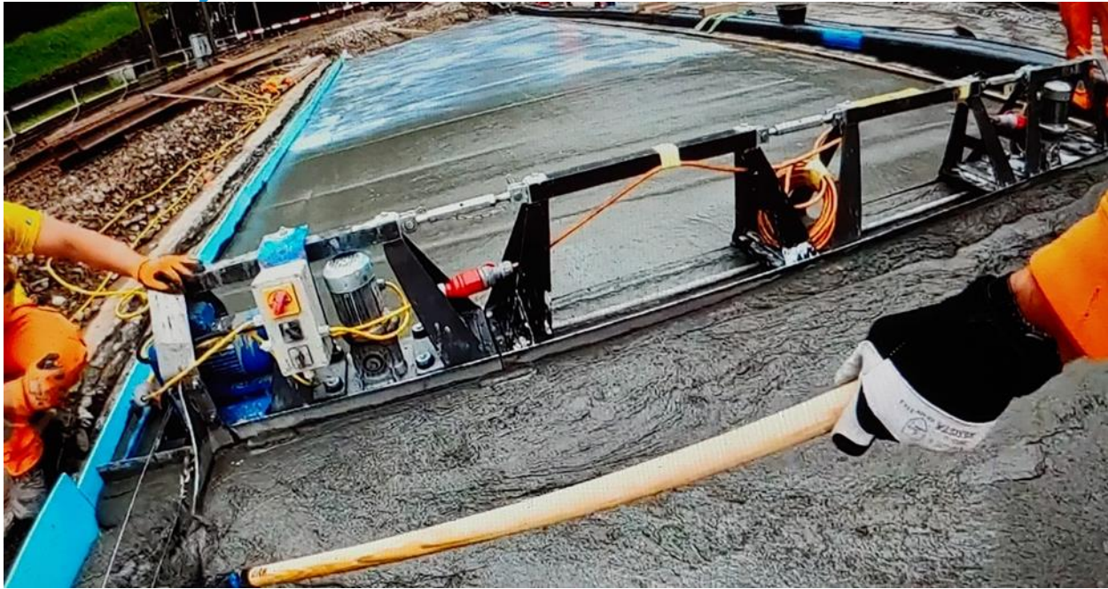
Photo: Placing ceEntek ce200SF-t™ thixotropic UHPC with a vibrating screed
