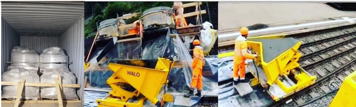
Photos: Container delivery of ce200SF-t™ Bulk-Bags (L); Batching of ce200SF-t™ and delivery in rail buggies on-site (R).
