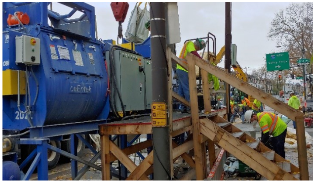
Photos: ceEntek's UHPC Mixers in pairs (L); Preparing to cast the connection between the PMUs (R).
