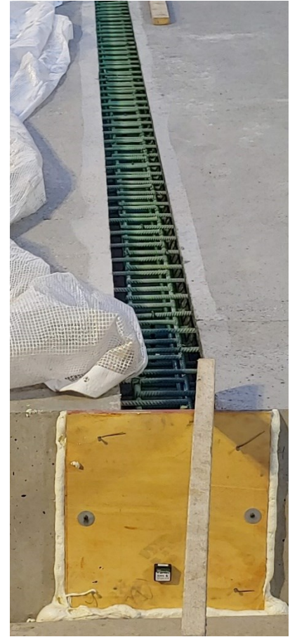
Photos: ceEntek's UHPC Mixers in pairs (L); Preparing to cast the connection between the PMUs (R).
