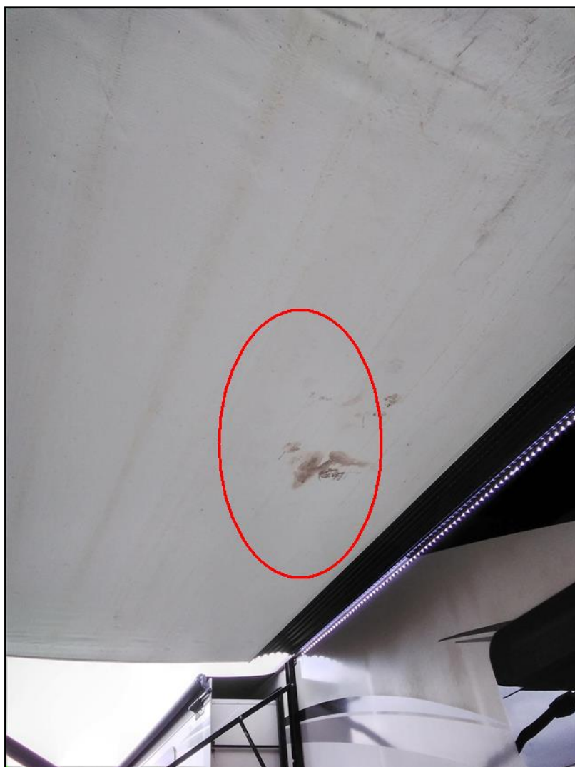
underside of awning
