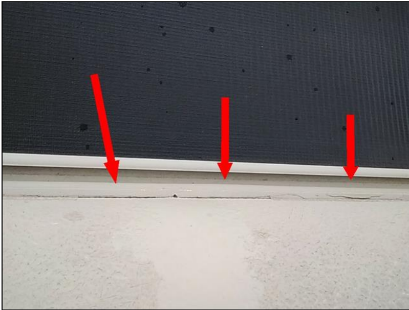
streetside gutter trim rail
