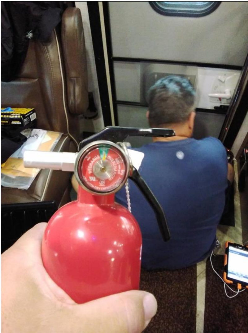
fire extinguisher gauge
