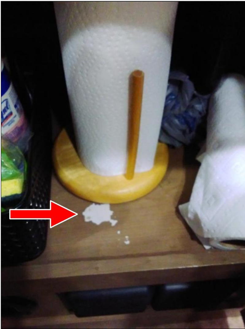
under kitchen sink
