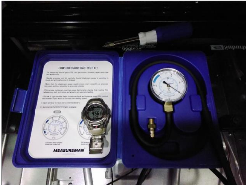
LP pressure test end
