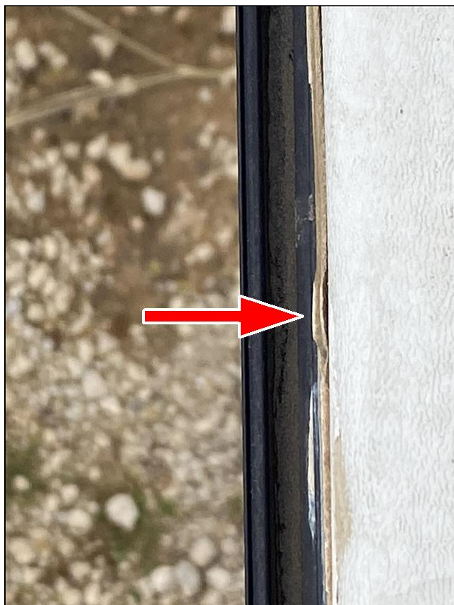
rear curbside gutter
