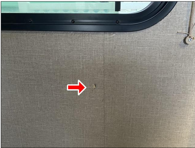
hole in wall
