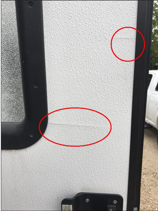
Cracks on interior main door
