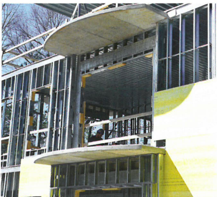
Cantilevered Formed-in-place Balcony
