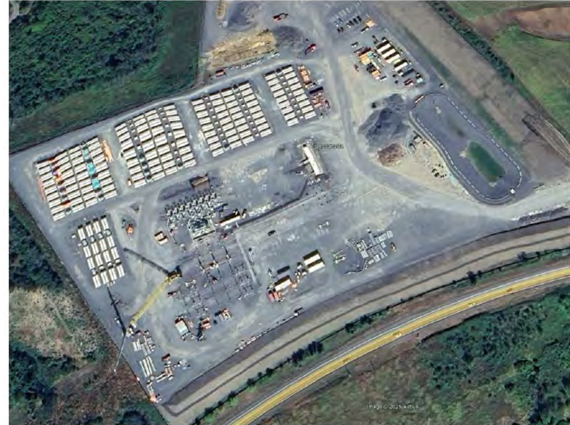
Atura/OPG Napanee Energy Centre Phase 1 Construction
