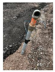
Standpipes, as shown above, have been installed in various locations to assist with the testing of the water main prior to it being placed into service
