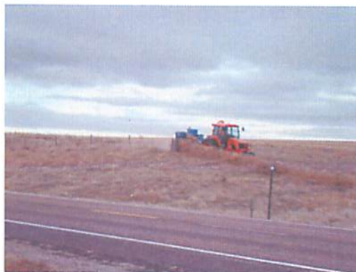
Fence line after cleaning
