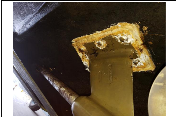
Bottom Prop Strut has had Maintenance
