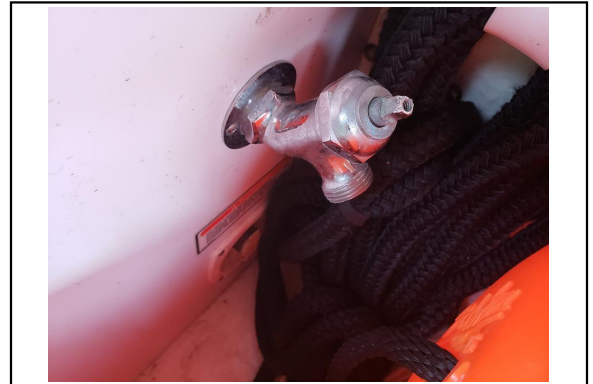
Water City Handle Missing
