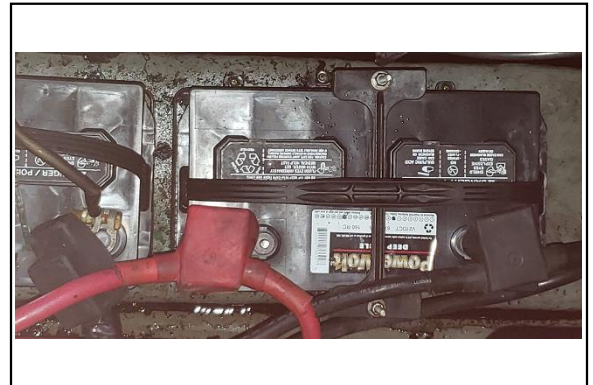
Battery + Terminals not Covered (2)
