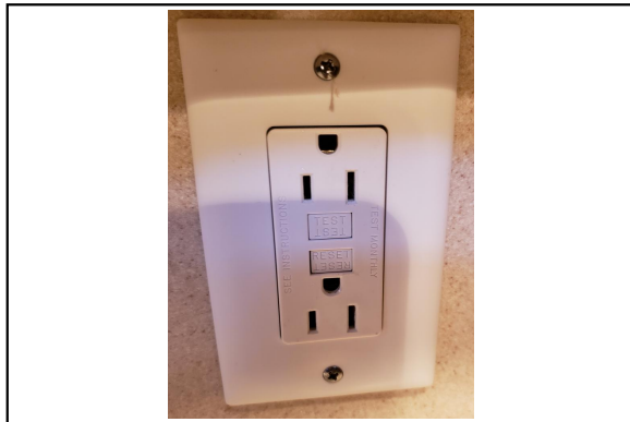
Electrical Outlets are GFCI
