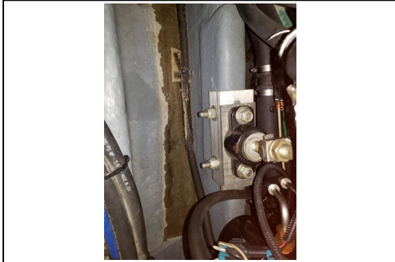
Bilge Water Standing
