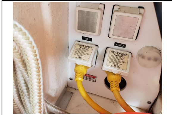
Shore Power Cables Two
