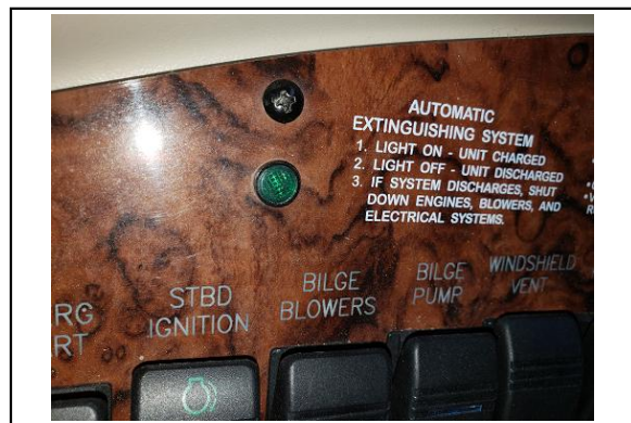
Helm Fire Extinguisher Shows Charged
