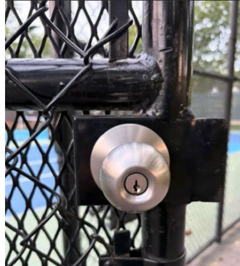
New Lock replaced
